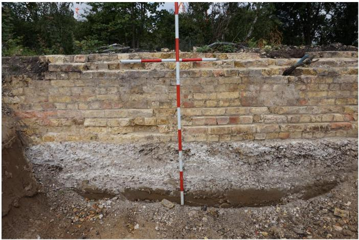
Plate 8: Looking west at exposed elevation of the foundation of the outer wall of the main building. Floor level would be at the top of the wall. Colour section of the scale is 0.2m long.
