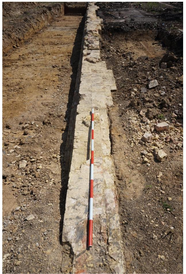
Plate 9: Looking south at west wall of the building and trench 9 and 10 accordingly on the left and right side of the wall. Outside of the building is on the right side of the wall. Wider sections of the wall are piers that were supporting arched lintels spanning over window bays.
