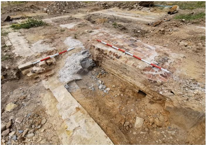
Plate 21: Looking north-west at room located within south end of east side building. Robust brick and concrete foundations were accommodating heavy machinery of some sort, very likely water compression pump. Possibly a wheel pit is located behind the structure [1509] with 2 metres scale bar. There is a leaver mechanism in the socket below right end of two metre scale. Grey concrete blocks visible
